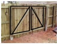
Each frame is a square measuring 4.5 m by 4.5 m with a diagonal support. The frames are highlighted in black in the picture above.
